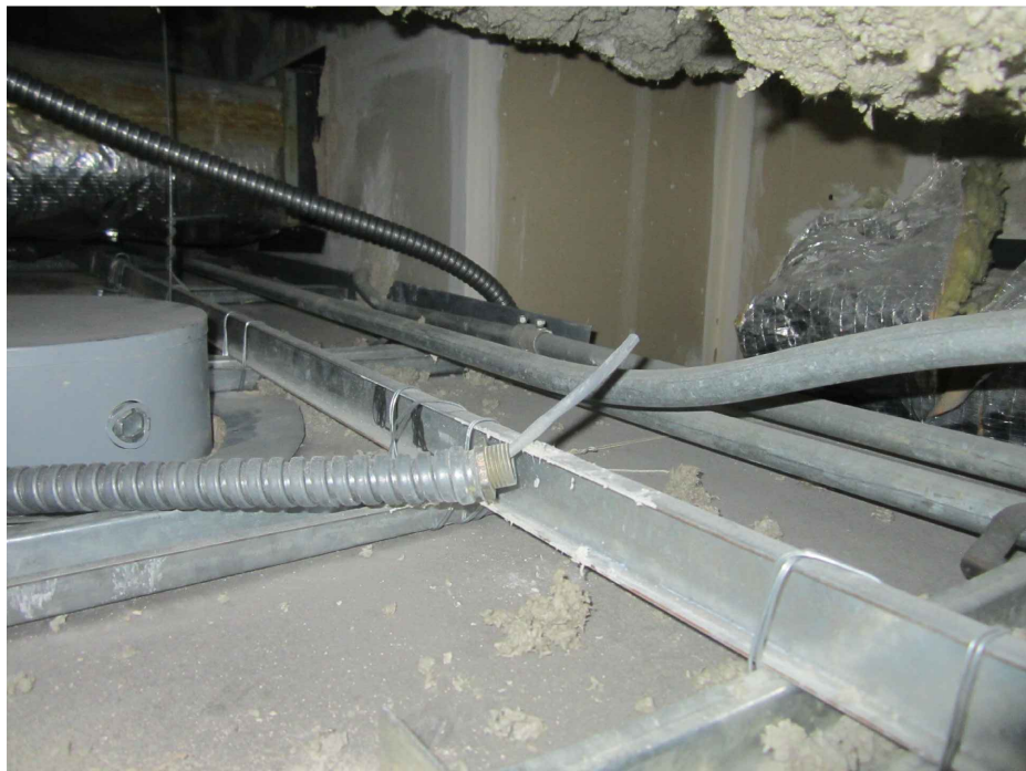
SPEAKER & CONDUITS AT CEILING (NORTH WALL)
