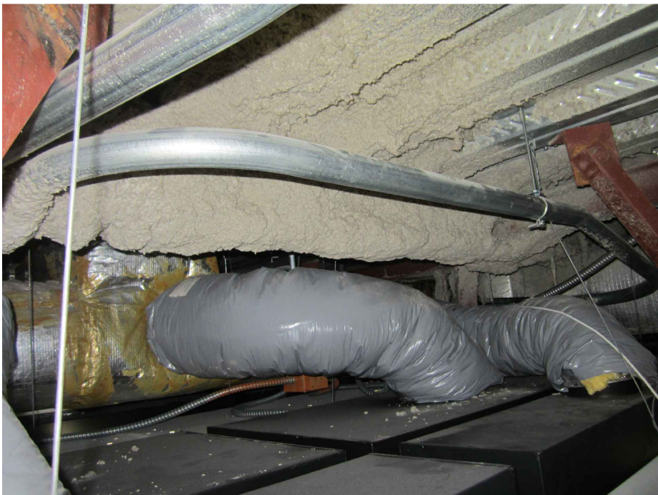
2"C AND MULTIPLE MISC CONDUITS AT CEILING
