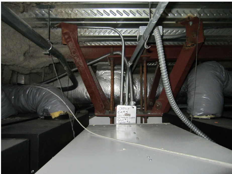
JUNCTION BOX & MISC CONDUITS AT BOOM SUPPORT
