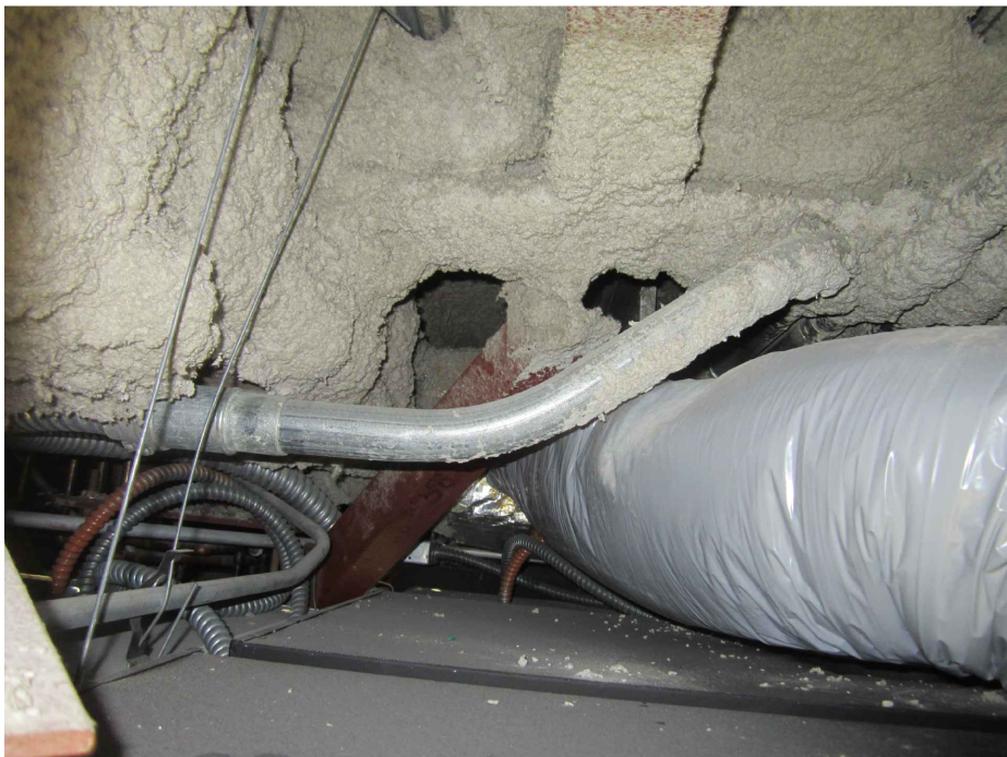
2"C AND MULTIPLE MISC CONDUITS AT CEILING
